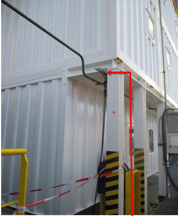
Figure 3 - Point A rigging
