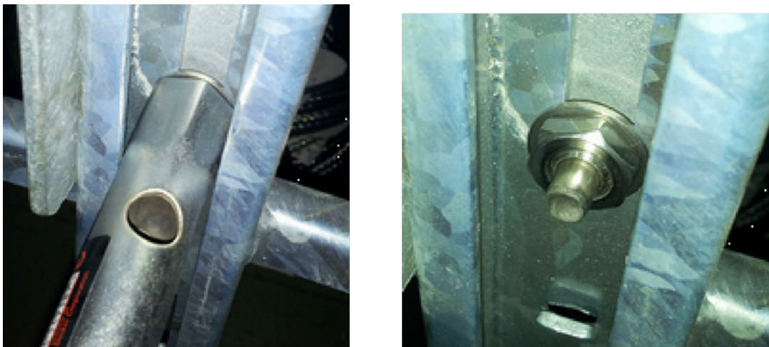
Figure 7: Assembly of nuts and installation position
